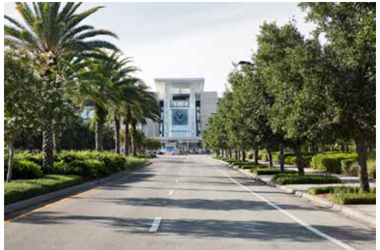
The New Orlando VA Hospital, part of the Medical City at Lake Nona. June 2014.
